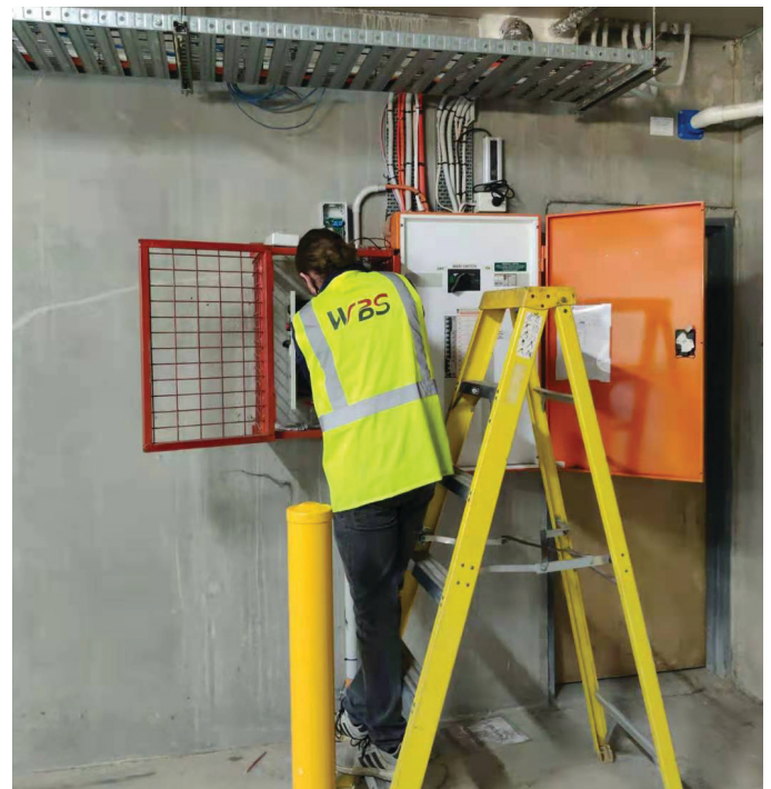
On-site installation being conducted by WBS Technology
